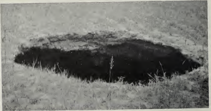
FIG. 19.—Cave-in on land south of Dewmaine where a 9-foot bed of coal is being mined at a depth of 100 feet. The opening is 12 feet in diameter and 15 feet below the surface; the width is approximately 25 feet. The hard pan arches up from the shale.
